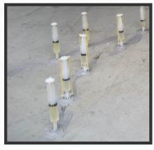
Our precision injection techniques effectively seal and repair structural cracks, preventing water ingress and restoring the integrity of concrete elements. We use epoxy, polyurethane, and cementitious grouts, depending on the specific project requirements.
